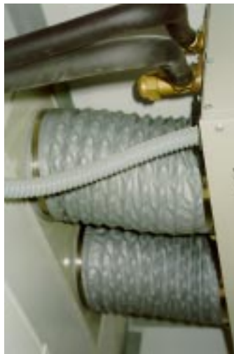
Fig. C – Freecooling ducts
