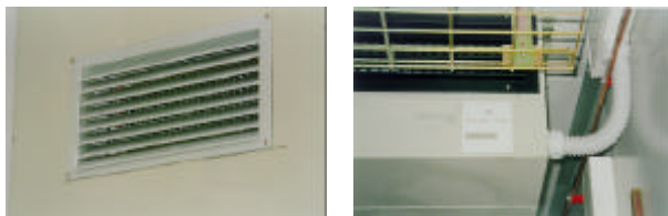
Fig. E – Internal overpressure damper with outside-oriented fin openings and its outside external waterproof protection grille.
