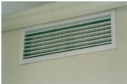
Fig. D – External inspectable rainproof grille with prefilter
