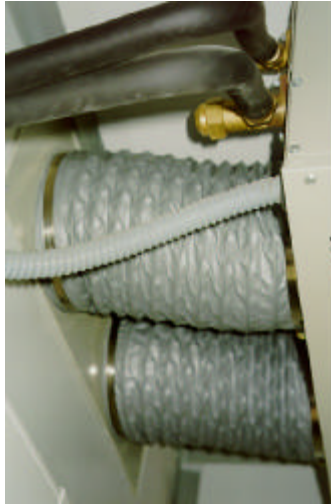
Fig. C – Freecooling ducts
