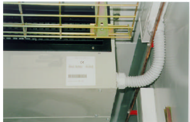
Fig. F – Details of the SE electrical connections with cable presser and plastic sheath (not supplied by us)
