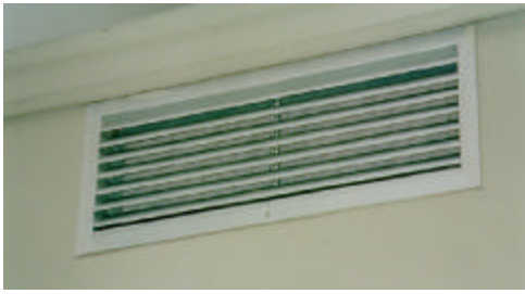
Fig. D – External inspectable rainproof grille with prefilter
