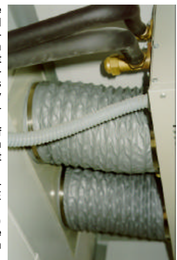
Fig. C – Freecooling ducts
