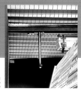
aluminium balanced 3-stage progressively operating, 3-phase, electric reheaters have a low surface temperature in order to avoid problems due to ionization.
