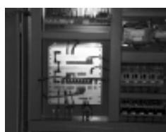
The components of both power and control are split into two sections of one panel. Individual key locked doors access each section, which prevents unauthorised entry. The panel is manufactured IP55 to ensure
