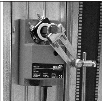
6 - Dampers prepared for actuator installation
