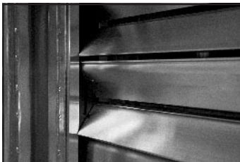
1 - Profile vanes of regulating damper
