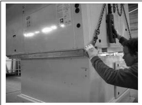
The baltic is moving down to the curb, the forklift protection are removed
