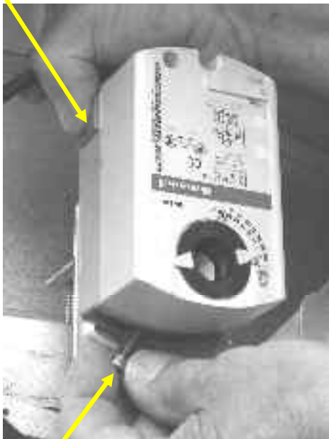
Manual rotation of the actuator
