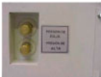
Pressure test point connections
